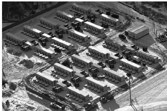
Figure 2 - Centrale inertielle de 20 MW, 2011, New-York, © Beacon Power.
